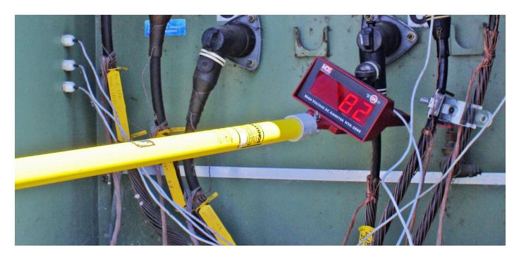
Primary voltage cables are generally shielded and the Ammeter cannot measure current on a shielded cable except in areas where the shield has been removed.
